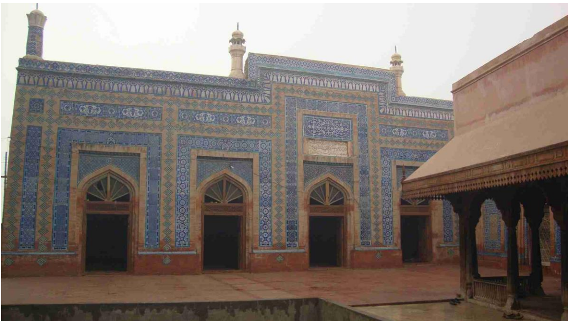
The Mosque adjacent to the Shrine of Saiyyid Jalal al-Din Surkh Bukhari
